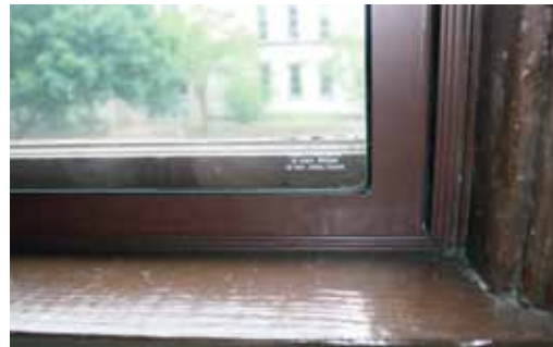
Recommended: [26] The new metal interior storm window was carefully matched to the exterior window as part of the rehabilitation of this historic armory building.
