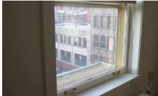
Recommended: [28-29] These exterior storm windows match the pane configuration of the historic interior windows in a residence and in a multi-story hotel building.
