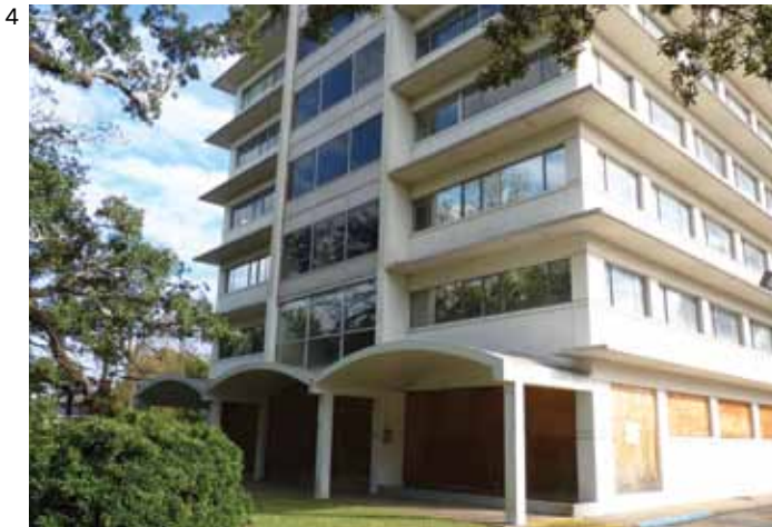
[4] Covered walkways and horizontal sun screens are distinctive and sustainable features in some mid-century modern office buildings.
