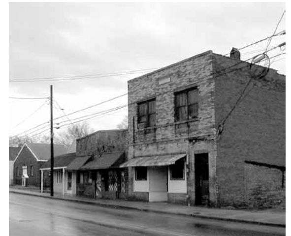
The Cansler Building at 1518 University is significant for its architecture, (a Commercial Vernacular style with distinctive brick work), its representation of African-American economic development, and its builder Charles W. Cansler, a noted African-American educator, entrepreneur and community leader. The building is being rehabilitated as part of Stephens Square, a portion of the Hope VI development, and is protected by an H-1 Historic Overlay adopted in early 2004.
