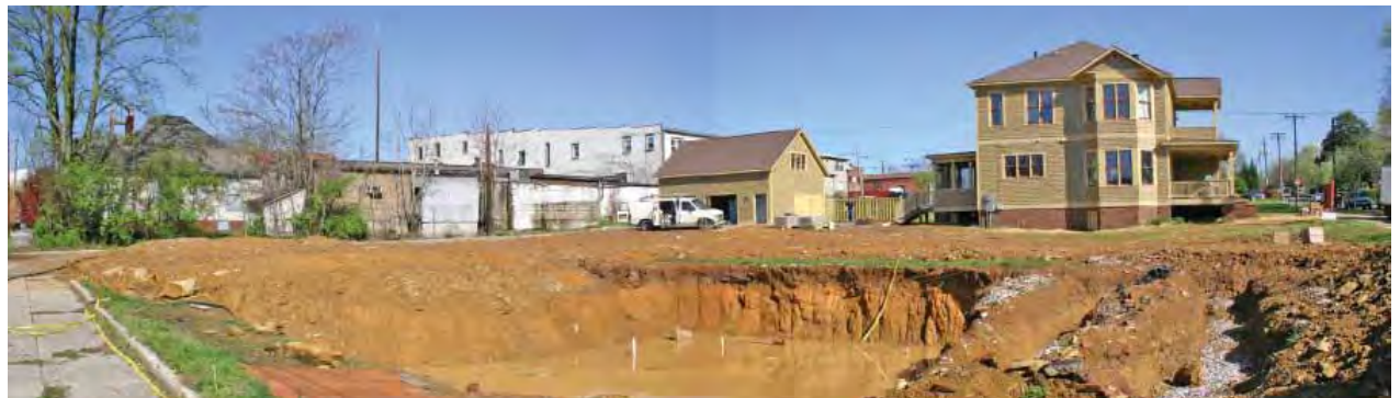
The success of neighborhood revitalization has begun to attract new construction to inner city areas. Pictured above are three lots in the 4th & Gill area. In the foreground footers have been laid for a new home; in the right background is a newly-constructed home that is near completion.
