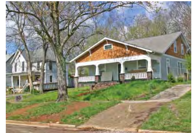
Two homes on Oklahoma Avenue are rehabilitated.
