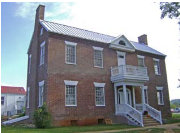
The Colonel John Williams house on Dandridge Avenue
