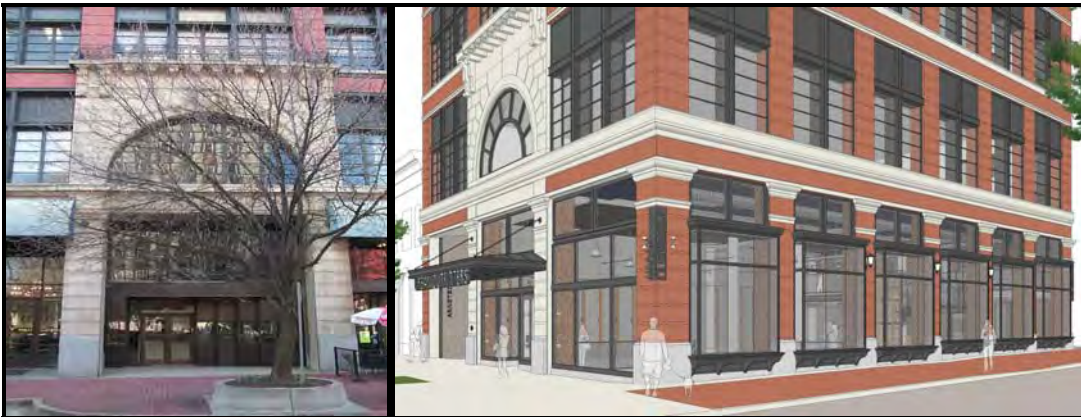
Arnstein Bldg. entry @ Market Street
