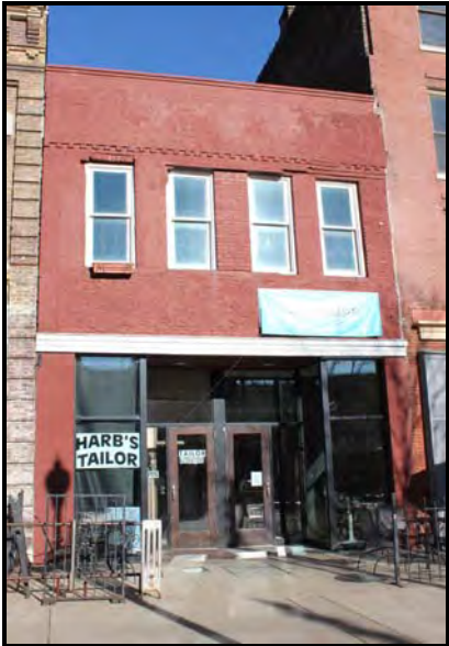
Second-level façade to be renovated at 32 Market Square
