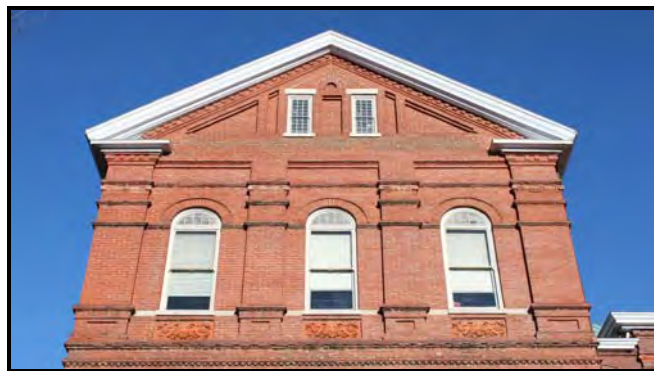
Upper level of County Courthouse facing west
