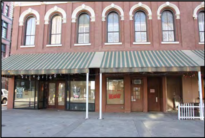
Storefront to be renovated for restaurant at 1 Market Square
